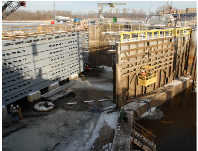
(Above: With bulkheads in place, work will be done on gates and walls in three Upper Mississippi locks)
