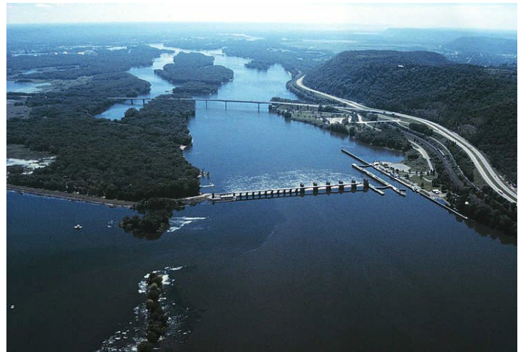
(Above) Lock and Dam 7 near LaCrescent, Minn., was one of the structures benefitting from stimulus funded repairs this past winter.
